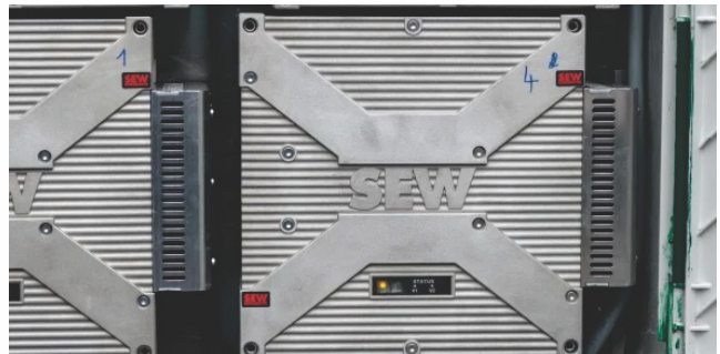
Four MOVITRANS® spot TES decentralized supply units
