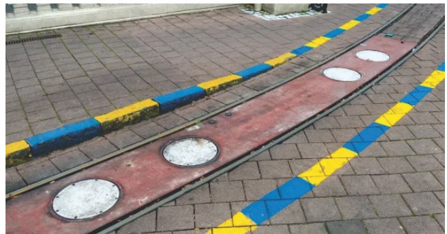
Stationary MOVITRANS® spot TFS field plates
