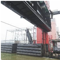
The troughs are sealed by sectional gates at the front and rear. Each of these lifting gates is raised by two individually driven segment chains that run along the machine house to the left and right of the gate.
