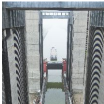
Each trough is suspended by 240 steel cables that run over pulley wheels housed in four towers
