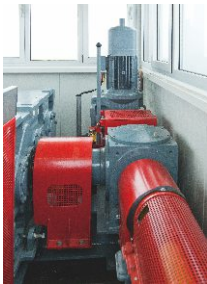
At the top is the industrial gear unit and auxiliary motor, with the transfer case and synchronization shaft below (from left)
