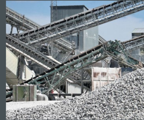
Cement production IE4 motors for distributing, conveying, grinding, and packing stone
