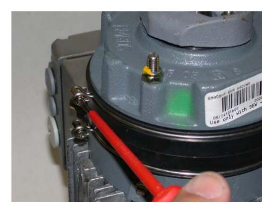
Remove the brake sealing band with the flat tip screwdriver, using caution not to damage the sealing band.
